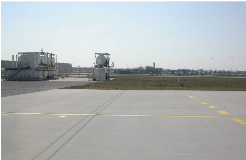
existing deicing tank farm at Leipzig Halle Airport
